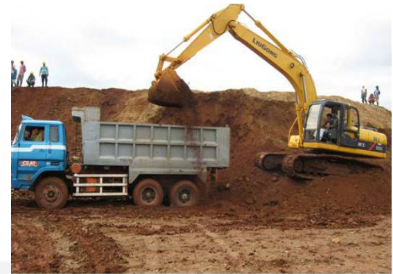
Stockpile Sorting and Loading
